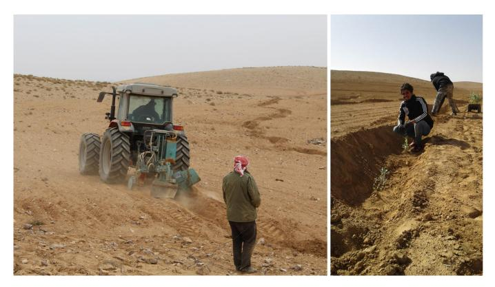
The Marab system was implemented in the floodplains of the watershed to temporarily store and redirect surplus runoff. This system allowed for flood irrigation of different areas by filling gullies, levelling seedbeds, and building bunds and spillways. Livestock in this dry area had better access to fodder thanks to the Marab system's ability to collect and store water, which allowed for the development of high-yield crops like barley.
